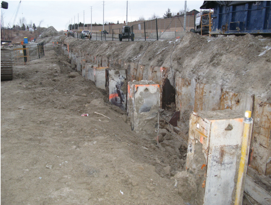
Figure 2. Section of proposed widened road with piles.
